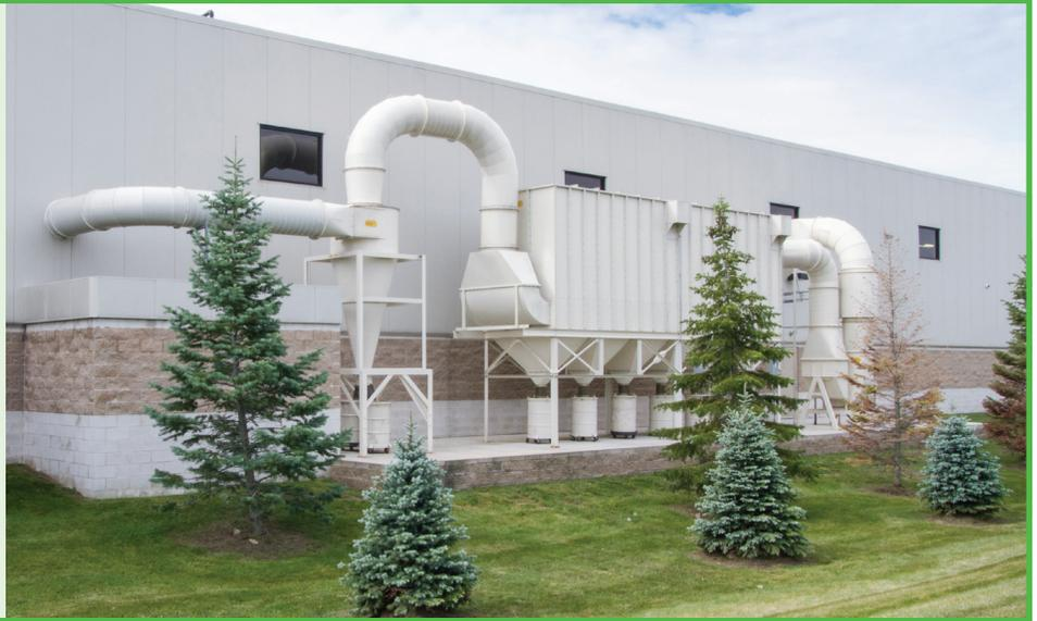
DUSTKOP collection equipment servicing a large school wood shop in downtown Detroit. Equipment includes a DUSTKOP 100N50-D2 cyclone unit primary dust collector with a 50 HP integral material handling fan, FH58-3 shaker-type after-filter, 5 HP scavenging fan re-inducing baghouse dust into the cyclone, and a DUSTKOP electrical control panel.
