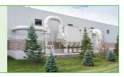
DUSTKOP collection equipment servicing a large school wood shop in downtown Detroit. Equipment includes a DUSTKOP 100N50-D2 cyclone unit primary dust collector with a 50 HP integral material handling fan, FH58-3 shaker-type after-filter, 5 HP scavenging fan re-inducing baghouse dust into the cyclone, and a DUSTKOP electrical control panel.
